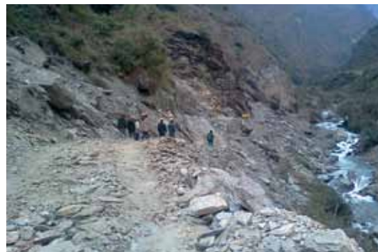
Access road construction in progress
