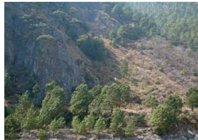
Under Ground Powerhouse site
