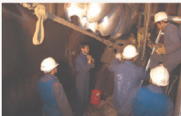
Nozzle Tip & Seat Ring Replacement (Annual Maintenance 2085)
