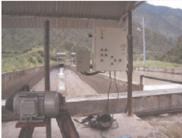
Motorization of Desander basin flushing gate
