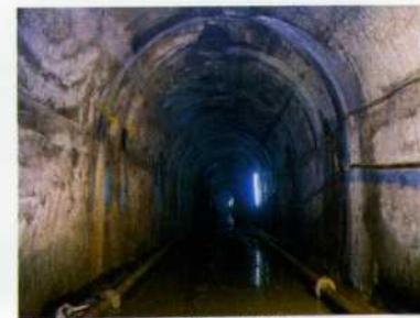
Headrace Tunnel (D-Shape Lining)
