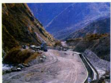
Open Power Canal
