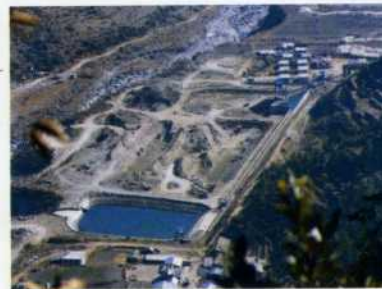
Partially Completed Reservoir
