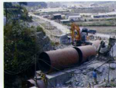
Steel Lined Pressure Conduit
