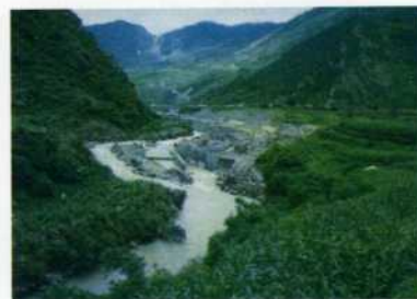
Headworks during construction
