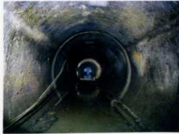
Headrace Tunnel (Circular Lining)
