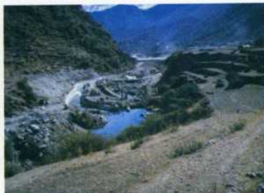
Headworks diversion during construction
