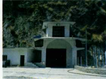
Access Tunnel to Powerhouse
