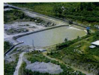
Partially Completed Reservoir Close View
