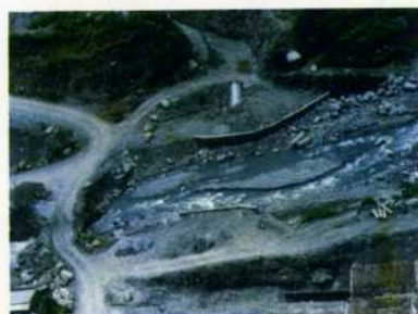
Syphon Beneath Bemdang Khola
