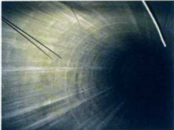
Surge Tank Looking Down
