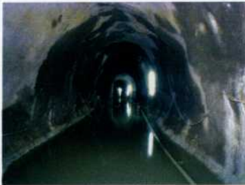
Headrace Tunnel (Shotcrete Lining)
