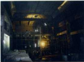
Underground Powerhouse during construction
