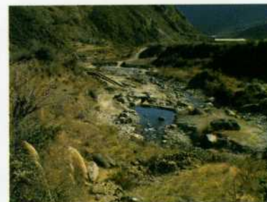
Bemdang Intake & Feeder Canal
