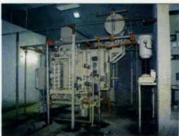
Single Phase Transformer
