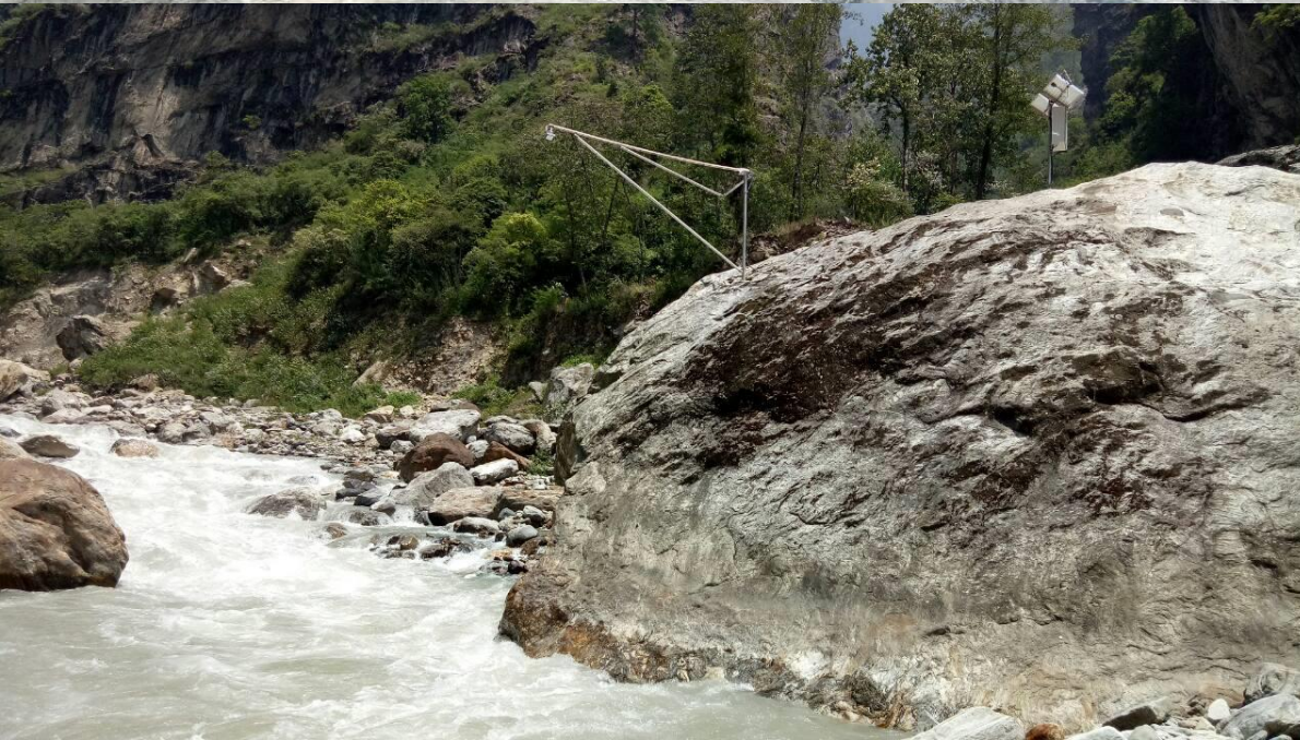
Automatic Gauge Station Setup near Lokpa
