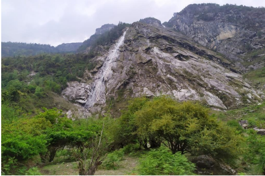
Rock outcrop of Banded gneiss in area of headrace inlet portal (Alternative 2(A), 3)
