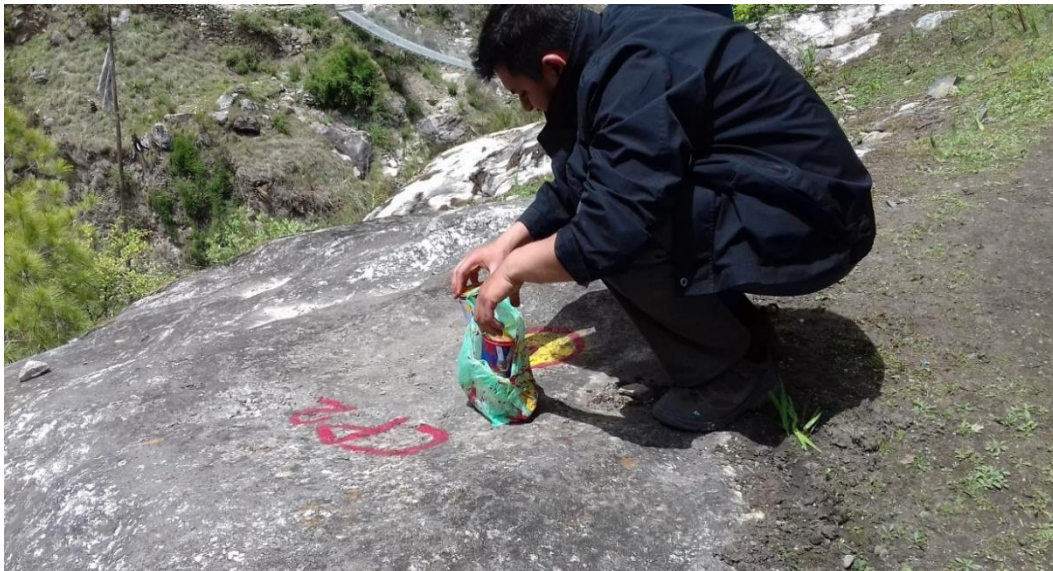
Monumentation of Control Point near Powerhouse location at Bihi
