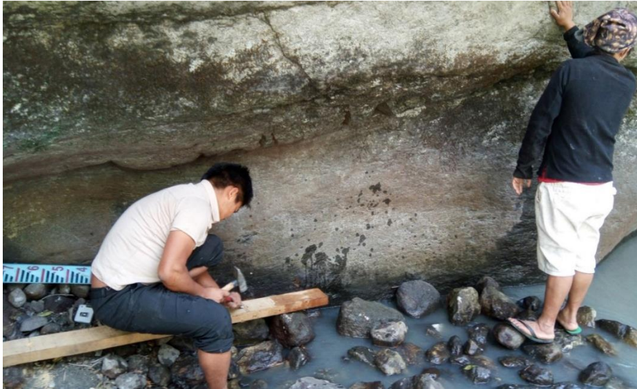
Installation of staff gauge u/s of Confluence of Budhi Gandaki River and Tom khola
